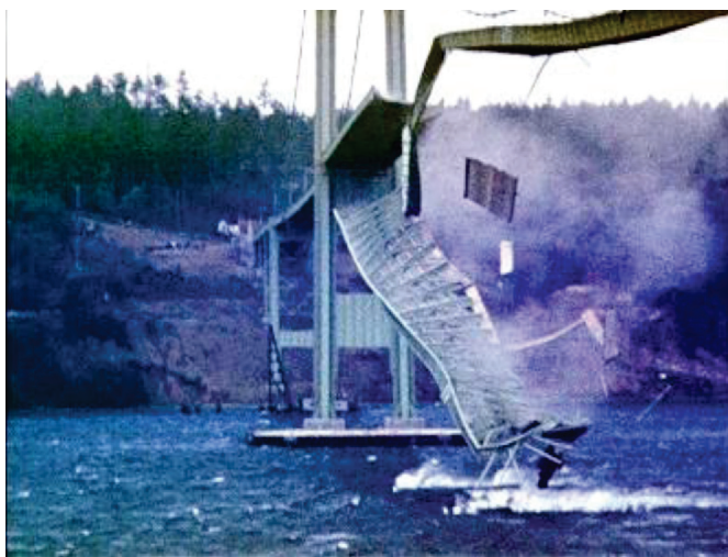
Fig.3-11; Vibrations breaking the bridge
